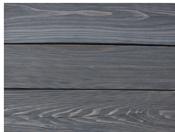
MONOGATARI - CYPRESS WEATHERED EXTERIOR INSTALL (NO TOP COAT REAPPLIED)
