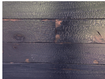
HAI - CYPRESS WEATHERED EXTERIOR INSTALL
