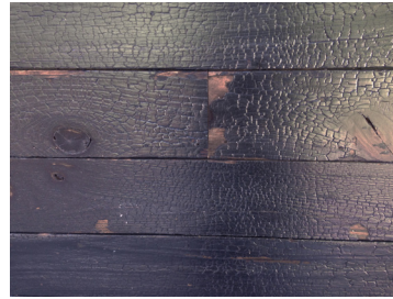
HAI - CYPRESS WEATHERED EXTERIOR INSTALL
