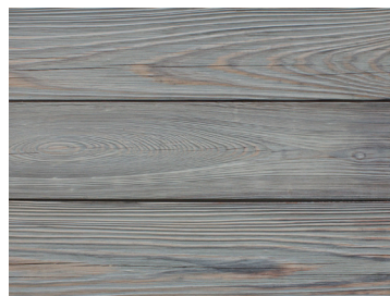
KUJAKU - CYPRESS WEATHERED EXTERIOR INSTALL
