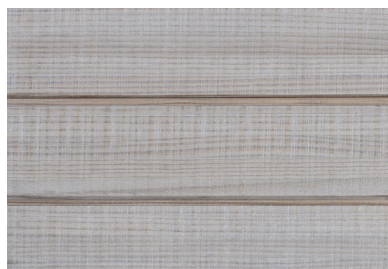
PATINA EXTERIOR CLADDING (WEATHERED 2 MONTHS)
