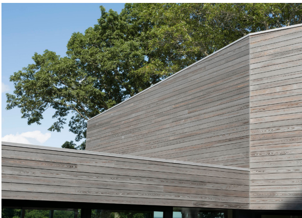
Charred Cypress cladding exhibiting natural tonal variation, visible grain contrast, and the evolving surface character associated with brushed charred finishes
