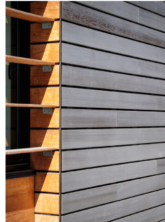
Western Red Cedar cladding exhibiting natural tonal variation and differential weathering associated with exposure, orientation, and moisture conditions; surface texture, grain pattern, and color evolution will vary across boards and over time
