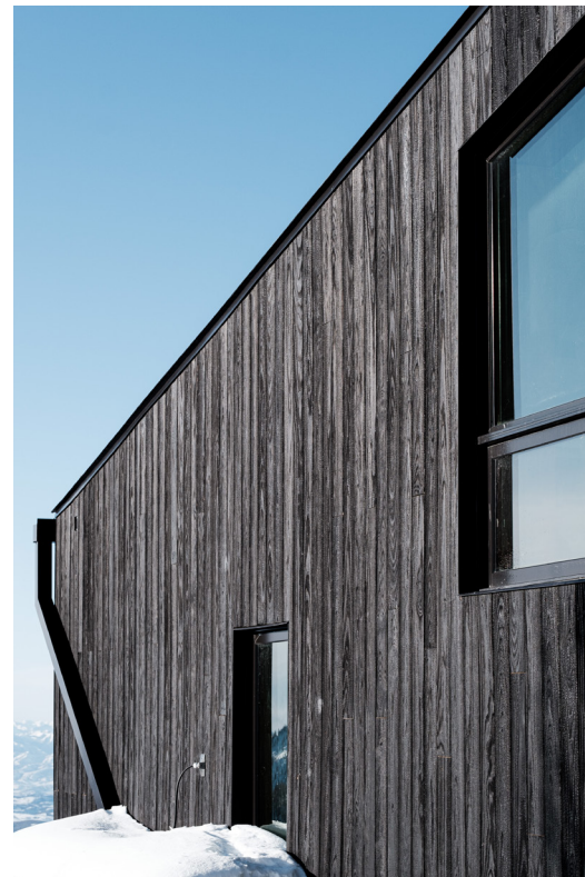
Charred Kebony® cladding exhibiting tonal variation, visible grain texture, and natural surface evolution associated with brushed charred finishes and exterior exposure
