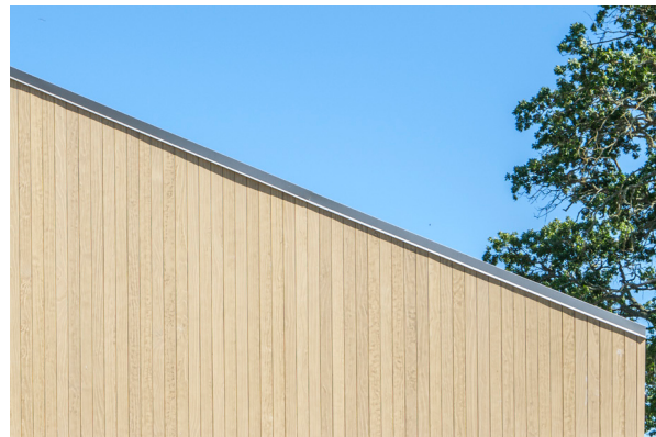
Prefinished Accoya® cladding exhibiting natural tonal variation, grain visibility, and board-to-board color shift inherent to modified wood products
