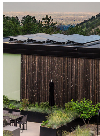
Charred Western Red Cedar exhibiting natural variation in char depth, grain exposure, and surface reflectivity; charred finishes will continue to evolve with exterior exposure and may weather differently across elevations and environmental conditions
