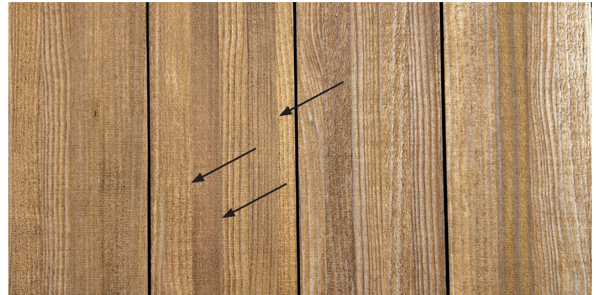
Example of laminated vertical grain Abodo Vulcan® cladding exhibiting natural tonal variation, grain reflectivity changes, and localized surface texture differences between laminated sections; variation of this nature is expected and does not indicate product failure or delamination
