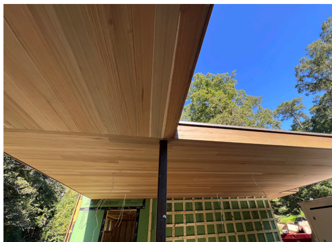
Alaskan Yellow Cedar exterior ceiling exhibiting natural tonal variation and grain contrast across boards; color variation, subtle sapwood presence, and shifting appearance under changing light conditions are inherent characteristics of natural wood products
