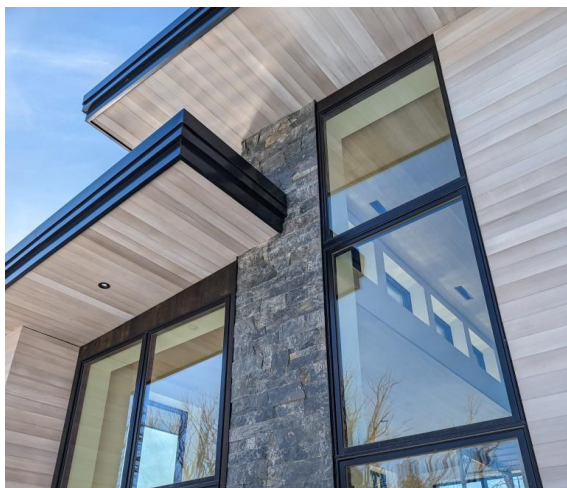
Clear Vertical Grain Alaskan Yellow Cedar exhibiting a refined linear grain pattern with moderate tonal variation; even within vertical grain selections, variation in color, texture, and finish absorption is expected and contributes to the natural character of the installation
