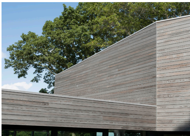
Charred Cypress cladding exhibiting natural tonal variation, visible grain contrast, and the evolving surface character associated with brushed charred finishes
